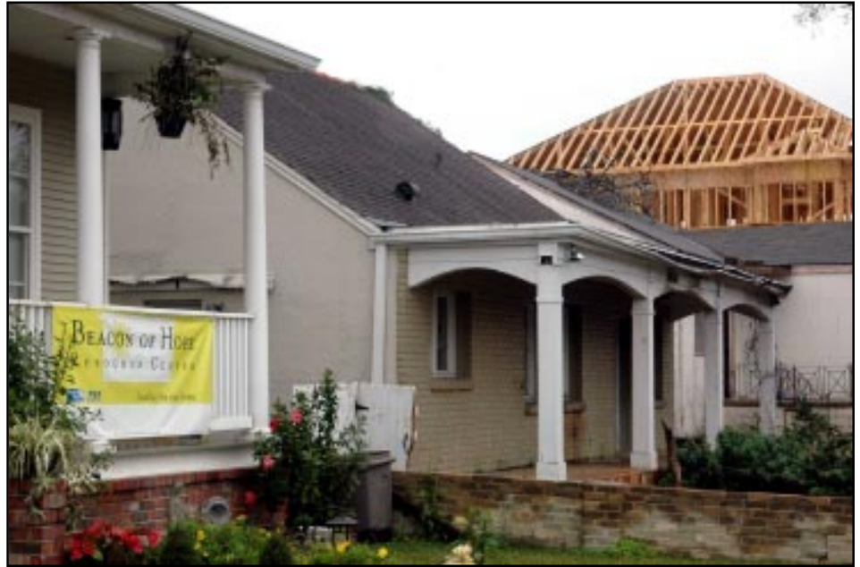
New construction fostered through the efforts of The Beacons of Hope program springs up amidst the lingering devastation.
