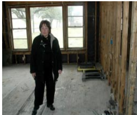
Linda Peppinger stands in what was once the living room of her Lakeview home. Linda and her husband John have not yet decided on what to do with the flood-ravaged structure.
